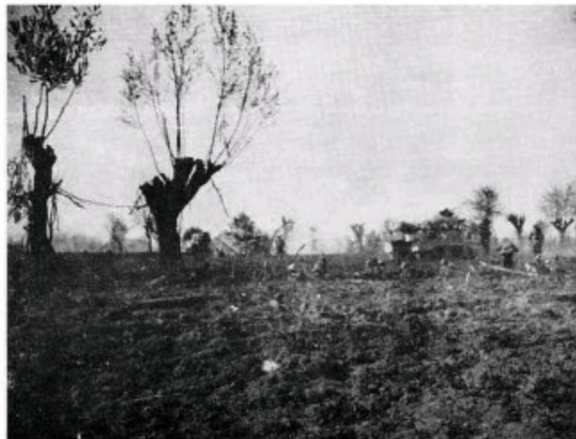
25 Battalion infantry and tanks advance towards the Santerno
