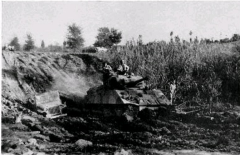
By-passing a demolition north of Rimini
