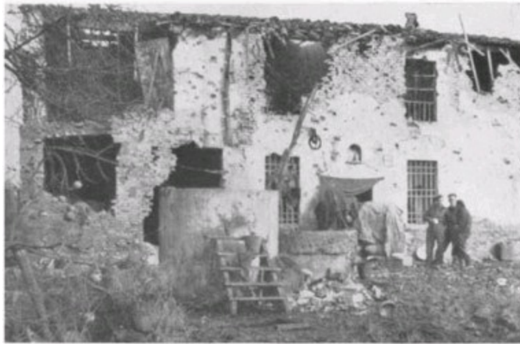
D Company headquarters, January 1945
