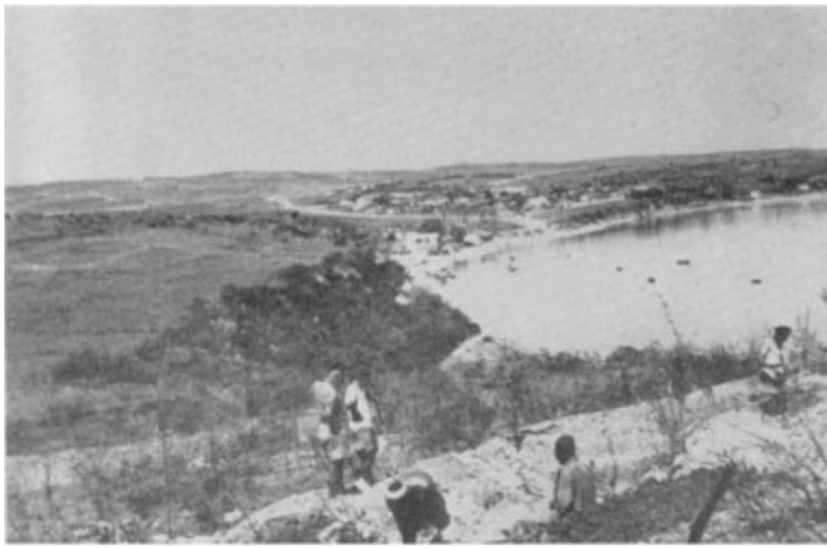
Digging defences on the Aliakmon line —Pal Elevation in the distance
