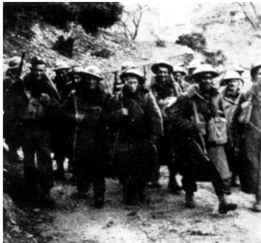
Climbing up the Monastery track from the Aliakmon River to the Pass road
