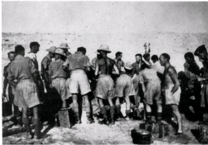
A burst pipe at the Qattara Box gave plenty of water for those with containers
