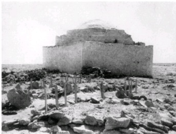
Sidi Rezegh mosque. New Zealand graves in the foreground
