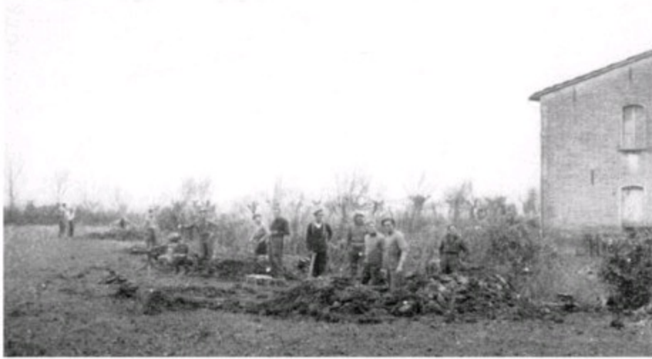
Digging in near Celle after 5 Brigade's attack
