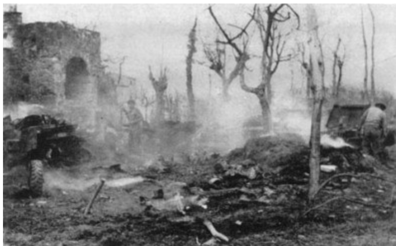
Route 6, about a mile from Cassino—a portée, two jeeps, and an anti-tank gun burnt out
