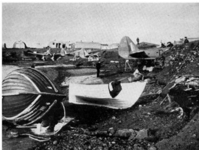
Aircraft at the edge of an airfield in Iceland protected from the high winds by mounds of earth and stones
