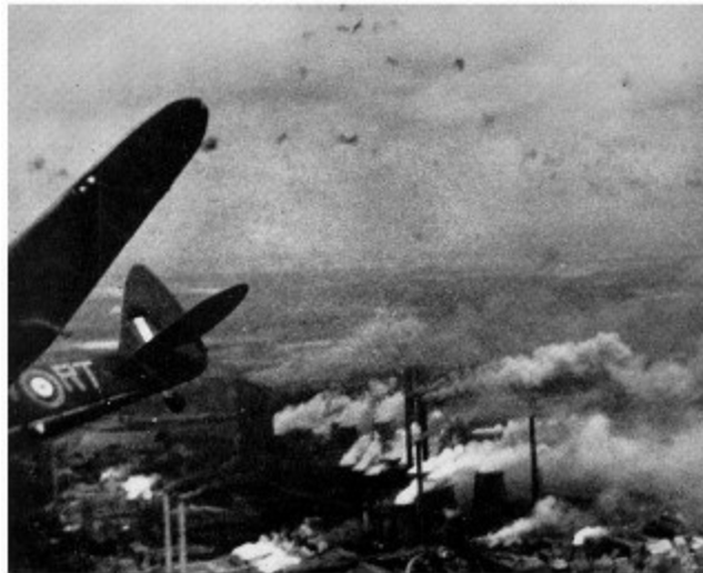
Attack on power stations at Cologne on 12 August 1941
