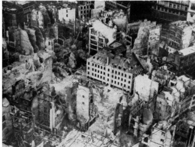
A section of London east of St. Paul's Cathedral after the raid of 29 December 1940
