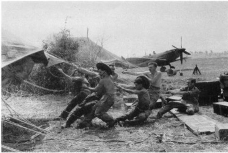
Ground crew of a Spitfire squadron in Burma erect a workshop during a minor monsoon
