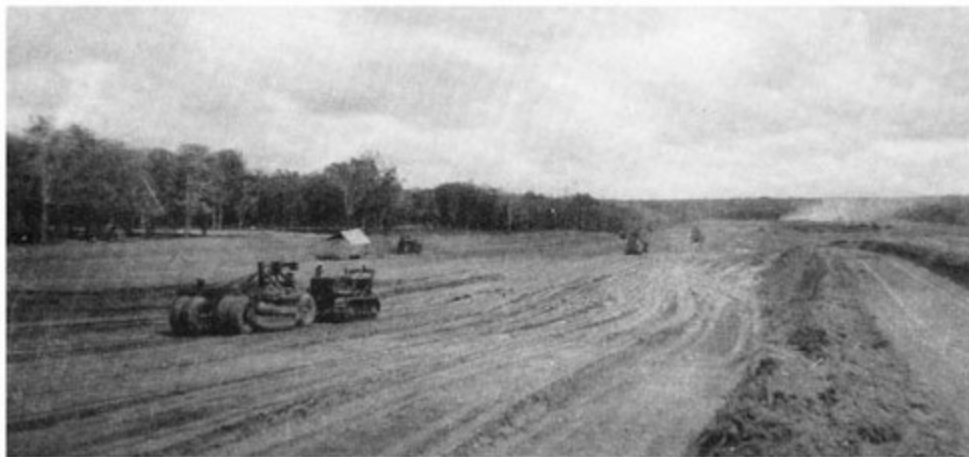
No. 1 Aerodrome Construction Squadron working on the bomber strip at Tebrau
