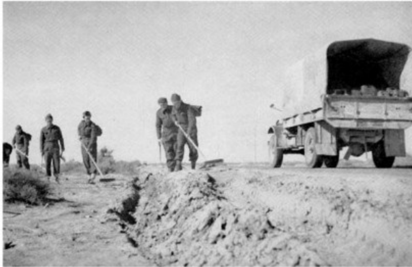
Engineers search the roadside for mines
