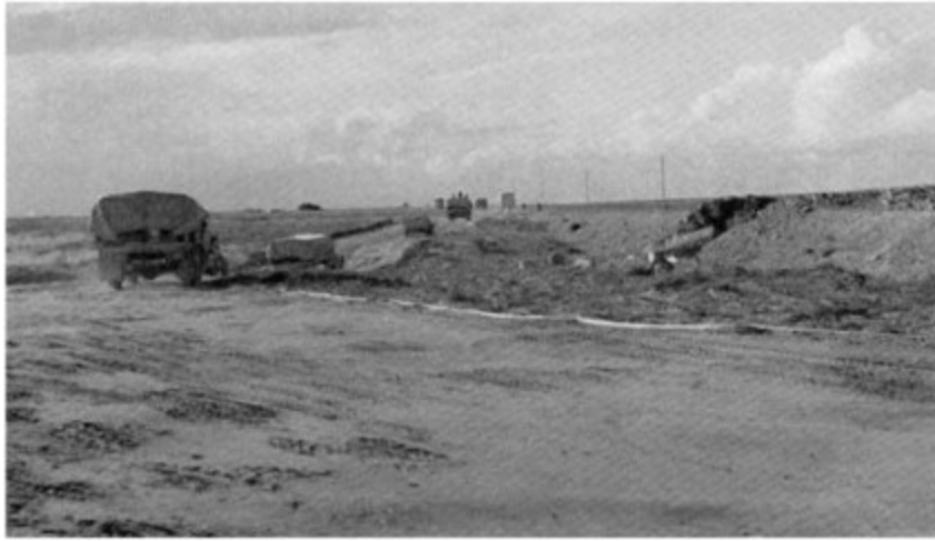
Bypassing a demolished bridge on the Via Balbia near Sirte . The white tape indicates the path cleared of mines
