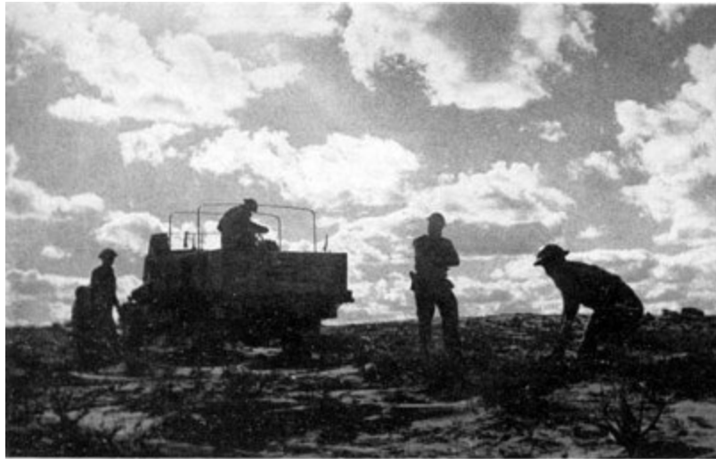
Laying a line from a cable truck
