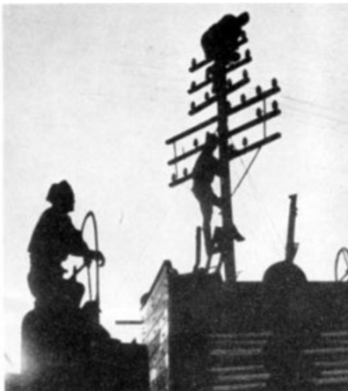
Repairing a bomb-damaged line
