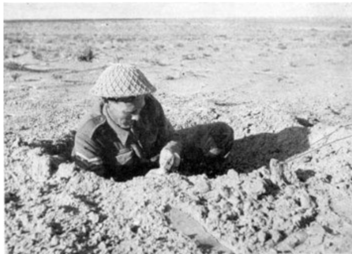
Repairing a line, Tripolitania
