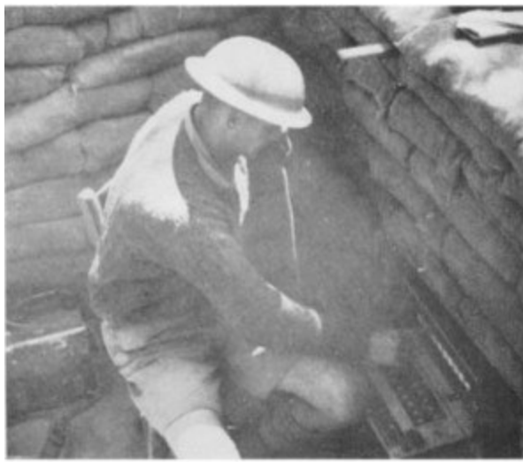
Divisional Headquarters' exchange at Galatas
