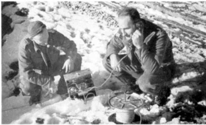
Testing field cable after the snowstorm on New Year's Eve 1943 — A. McKeachie and R. J. McConway
