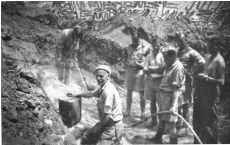
Sappers digging a gunpit, Syria
