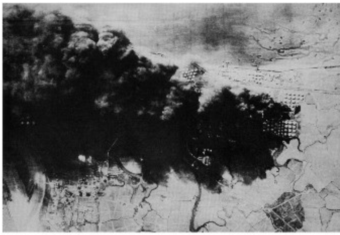
DAMAGE BY RAIDERS A photograph taken from a German aircraft of the enemy attacks on oil storage tanks at Newhaven on the Thames on 7 August 1940
