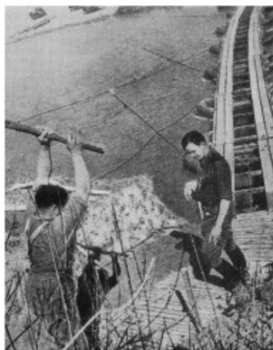
Pontoon bridge across the Pinios built by German engineers
