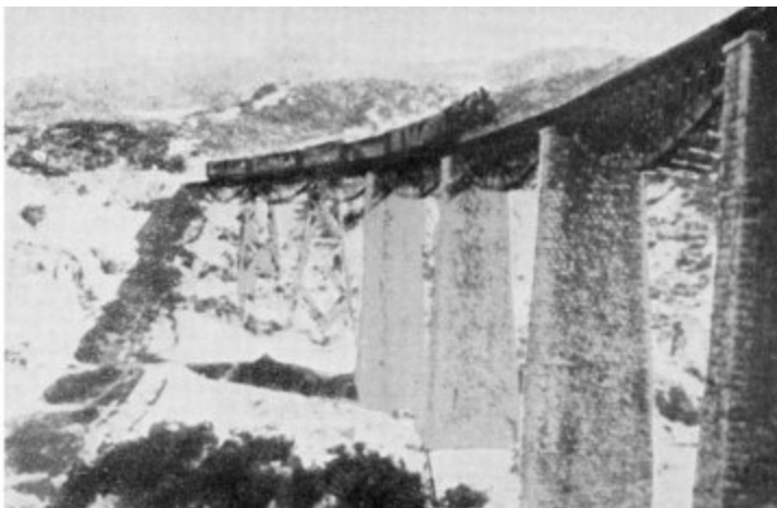
The Simplon-Orient express on the Gorgopotamos viaduct. The saboteurs used this photograph which, with the print below, was the only information available before the operation
