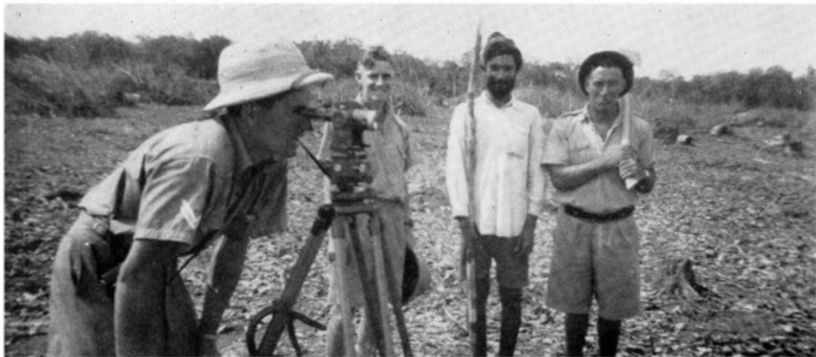
Surveying for a bomber aerodrome at Tebrau, Southern Johore
