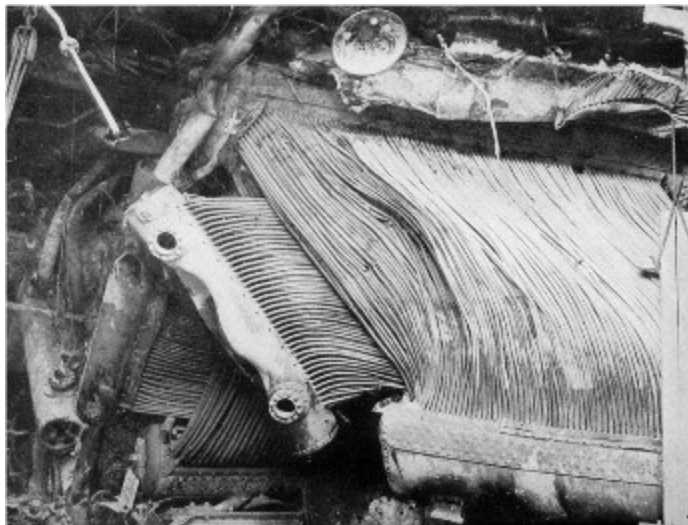
DAMAGE TO A BOILER CAUSED BY A JAPANESE TORPEDO
