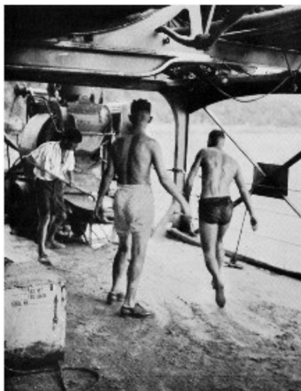
After Kolombangara, Cement was mixed for temporary repairs to the Leander . This photograph was taken near Tulagi Beach.
