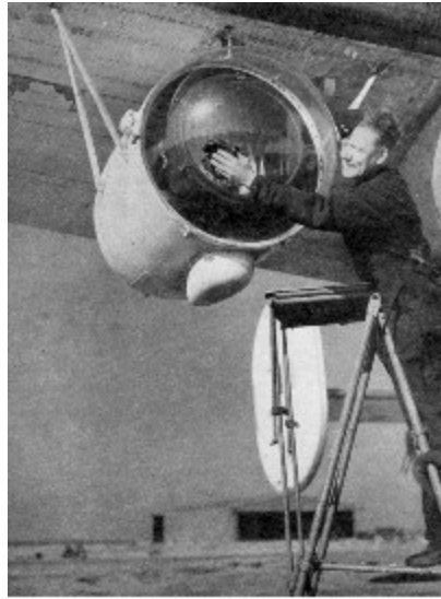
LEIGH LIGHT FITTED TO WING OF LIBERATOR
