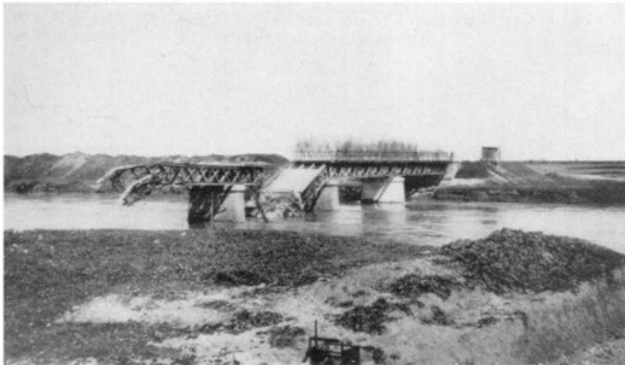
Blown bridge over the Aliakmon River
