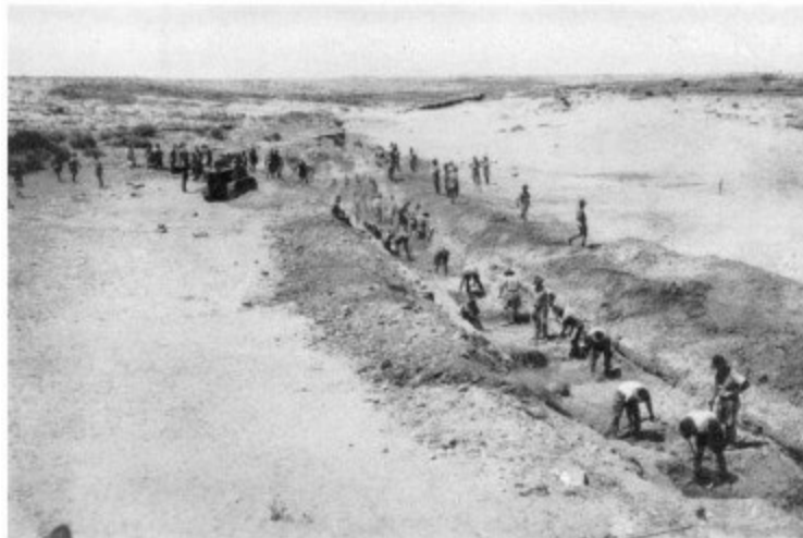
19 Battalion at work on the anti-tank ditch at Wadi Naghamish, June 1940
