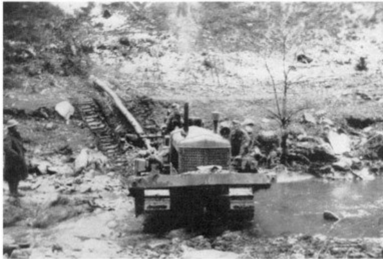
New Zealand engineers build a road in the Olympus Pass
