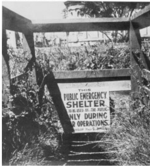
Entrance to an air raid shelter in Parliament grounds
