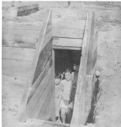
An air raid shelter under construction, Auckland, April 1942
