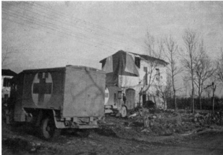
5 ADS, used during the attack on Faenza, December 1944
