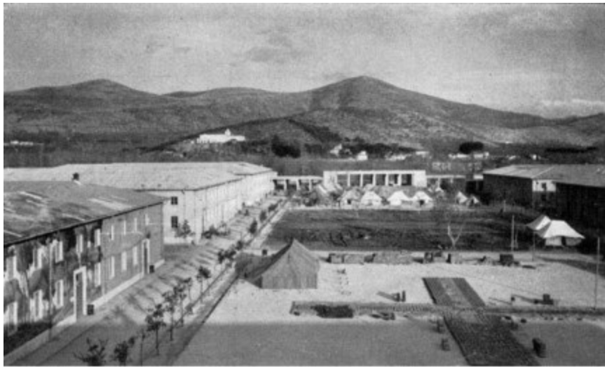
2 NZ General Hospital, Caserta, February 1944
