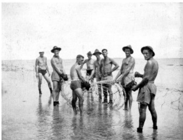
II NZ INFANTRY BRIGADE DEFENCES ON FIJI Wiring at low tide on Suva waterfront
