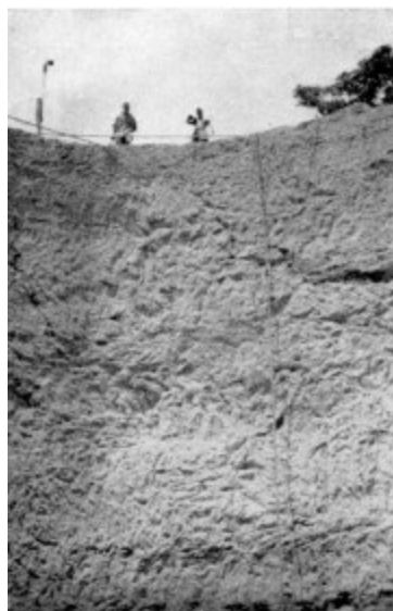
FACE OF PETROL TANK SUNK IN SOAPSTONE OF SEALARK HILL ,
