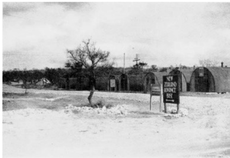
Main entrance to New Zealand Advanced Base, Taranto, March 1944
