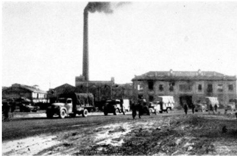
Supply Point at Forli Supply Point at Forli
